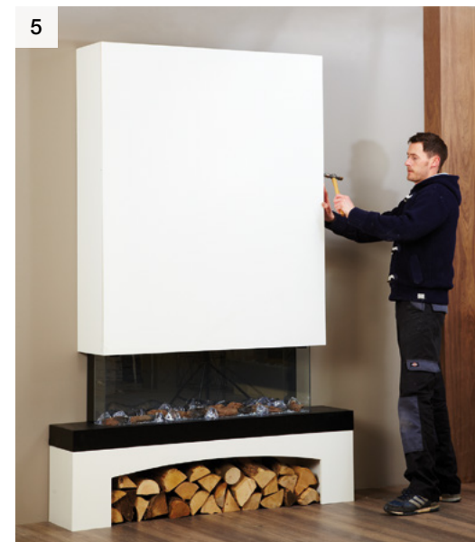
To finish. Use a fine nail punch to sink the pins below the surface. Then apply a small amount of Pollyfilla to fill the joint and the pinholes.
