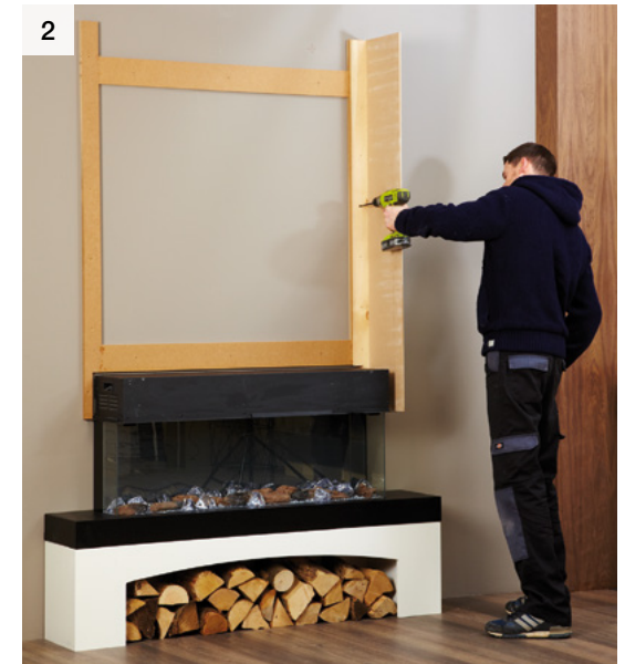
The right hand panel is then fixed onto the support frame by screwing through the pine batten.
