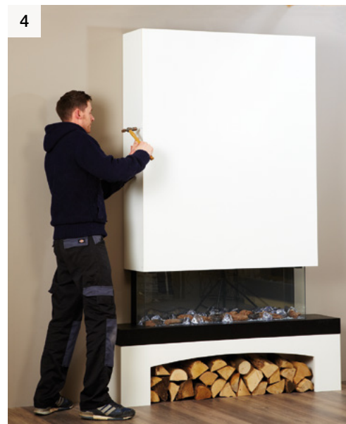
The front panel is fixed in position with panel pins. These are nailed through pre-drilled holes in the side panels.
